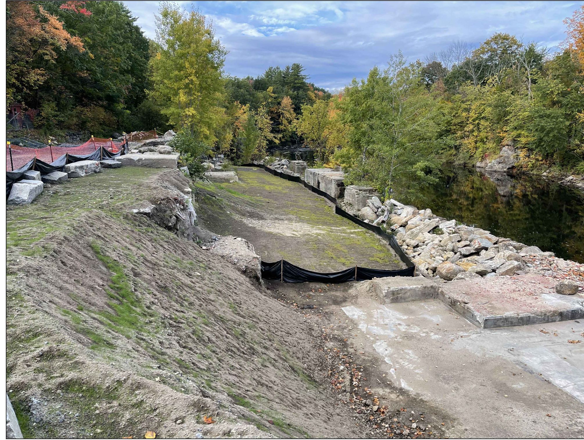
FORMER MILL SITE
