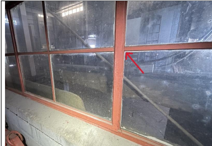
3. ACM HG5 Window Glaze in former exterior window
