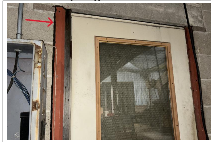
4. ACM HG10 Black Door Frame Caulk on former exterior door.
