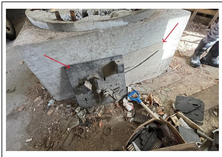
3. ACM HG102 & 103 – “Transite” Panels used as electrical backer boards and similar.
