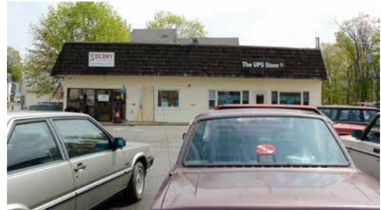
Existing facade of the Volvo building
