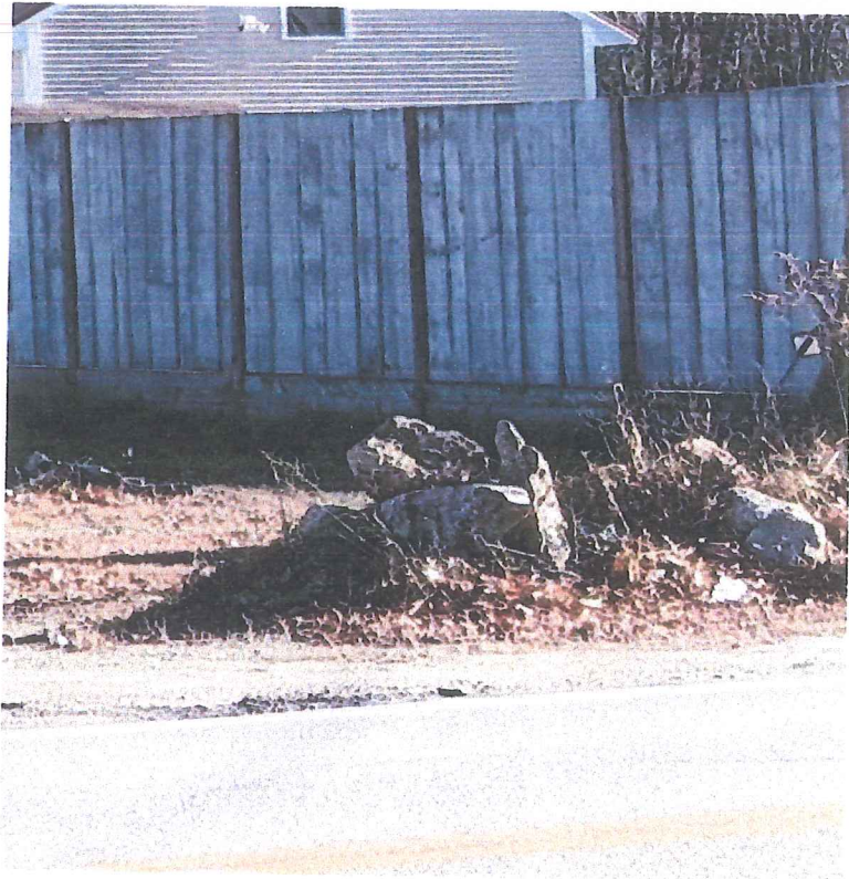
Two styles of unacceptable fencing (chain link and stockade)
